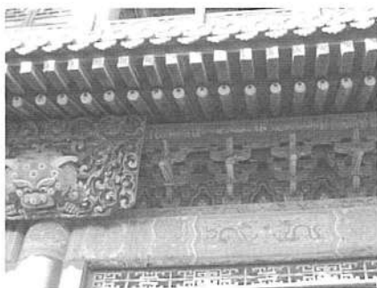
Fig. 5 a. The bracketing system in the east side of the three-tiered stage the Pleasant Sound Pavilion. Photo taken by Sasiporn Petcharapiruch on November 11, 2004.
